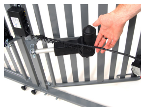
Ensure the power cable runs underneath the actuator
